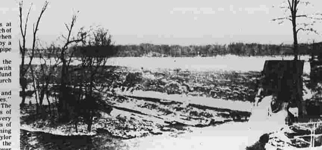
The Union Pond dam could once again begin generating electricity by as early as 1986 under a plan by a New York City-based company to build a generating plant on the dam in a partnership with the town. The town has been ordered to repairs to the dam, and revenues from the plant could be used to help defray the cost of the repairs.
