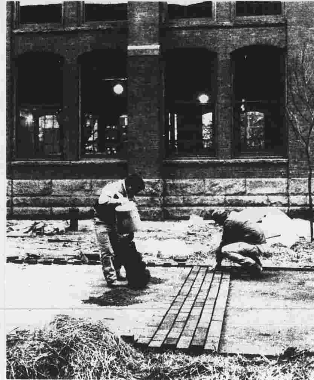
Mill becoming apartments Don Livesey (left) and Dave Cook, workers for Greenlee Landscape Co. of Bolton, lay brick for a sidewalk in front of the Ribbon Mill Apartments, which are under construction on Pine Street. Work is progressing on the 102-unit apartment complex being developed in the former Cheney mill in the historic district. New windows have been installed in the building, which formerly housed the Manchester Modes garment factory, and a new parking lot has been built.
